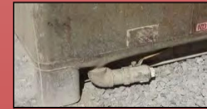
Screw Off Elbow Increases Chance of Leaking
